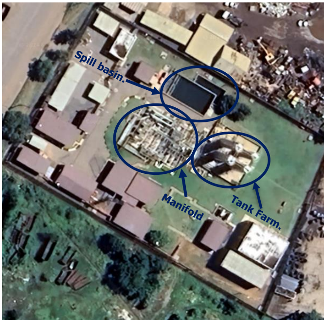
Figure 2: Spill Basin, Manifold and Tank Farm Arial View
