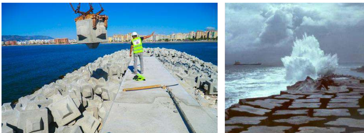
Figure 5-8: Example of Cubipod (left) and Antifer Block (right) armouring systems (Medina & Gomez-Martin, 2016), (Frens, 2007)
