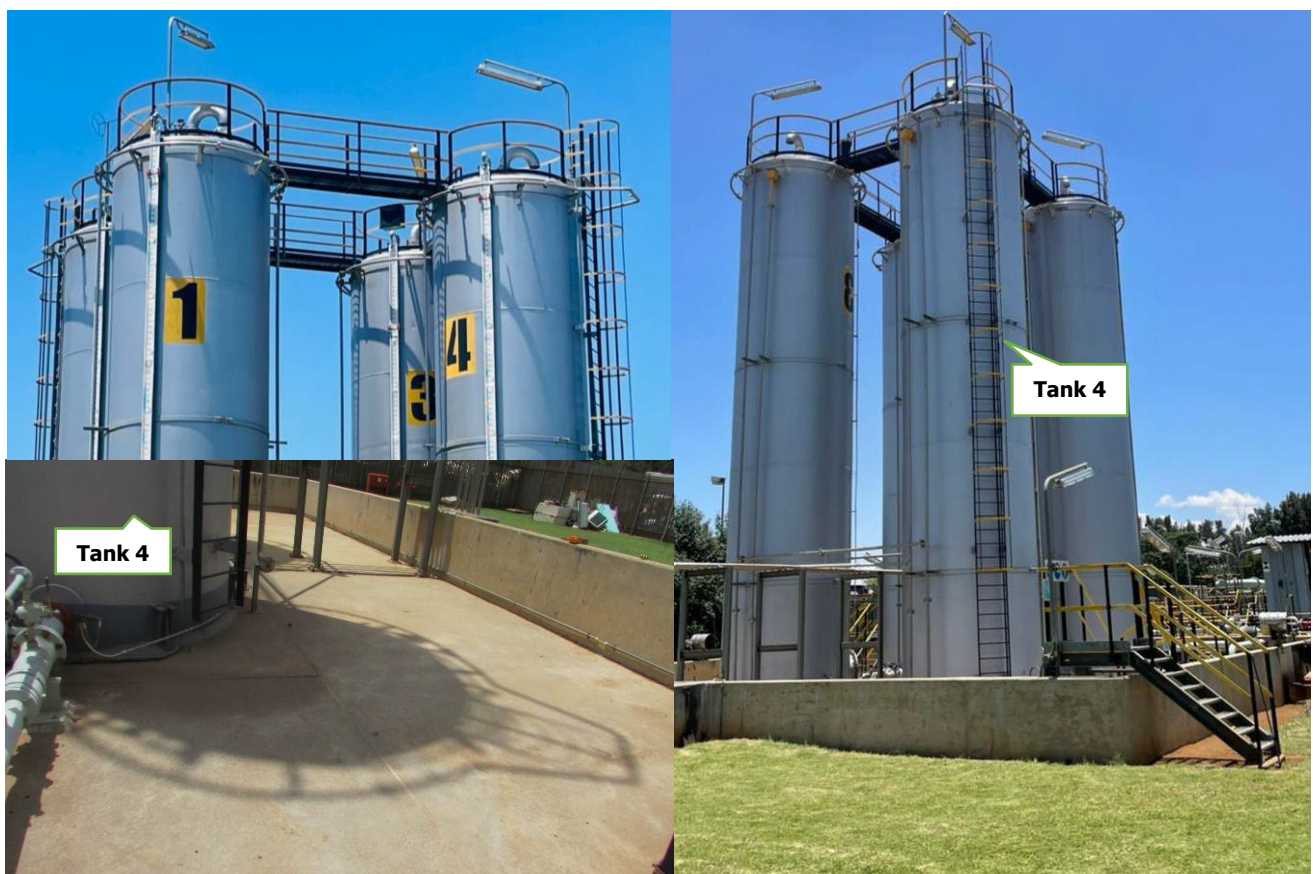
Figure 1 Klerksdorp Depot Intermixture Tanks: Left Top: Tanks numbered 1-4, Bottom Left: Space within bund wall, Right: Existing cat-ladder on tank 4
