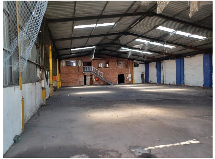
Figure 3-4: Interior of Warehouse 2.
