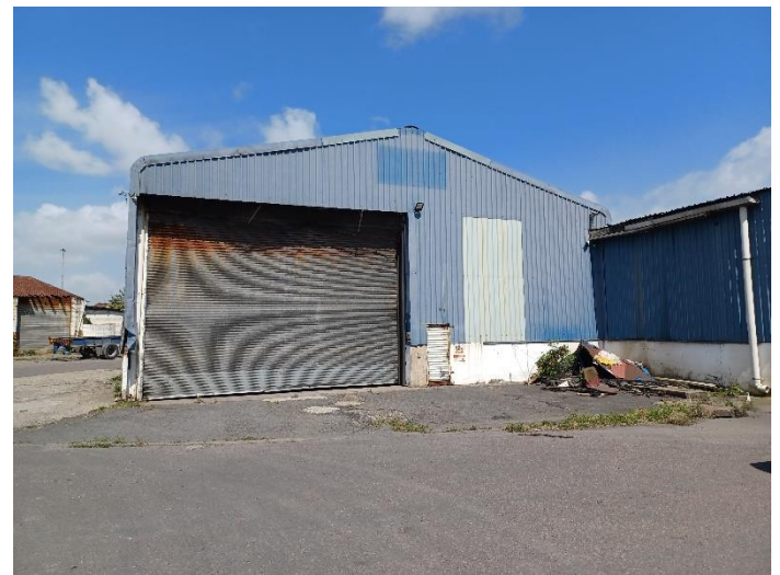
Figure 3-2: Exterior of Warehouse 1.
