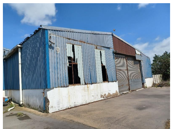
Figure 3-3: Exterior of Warehouse 2.
