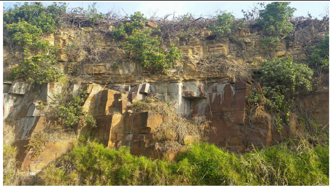
Photo 2: Horizontal bedding planes showing signs of groundwater percolation below weathered zone
