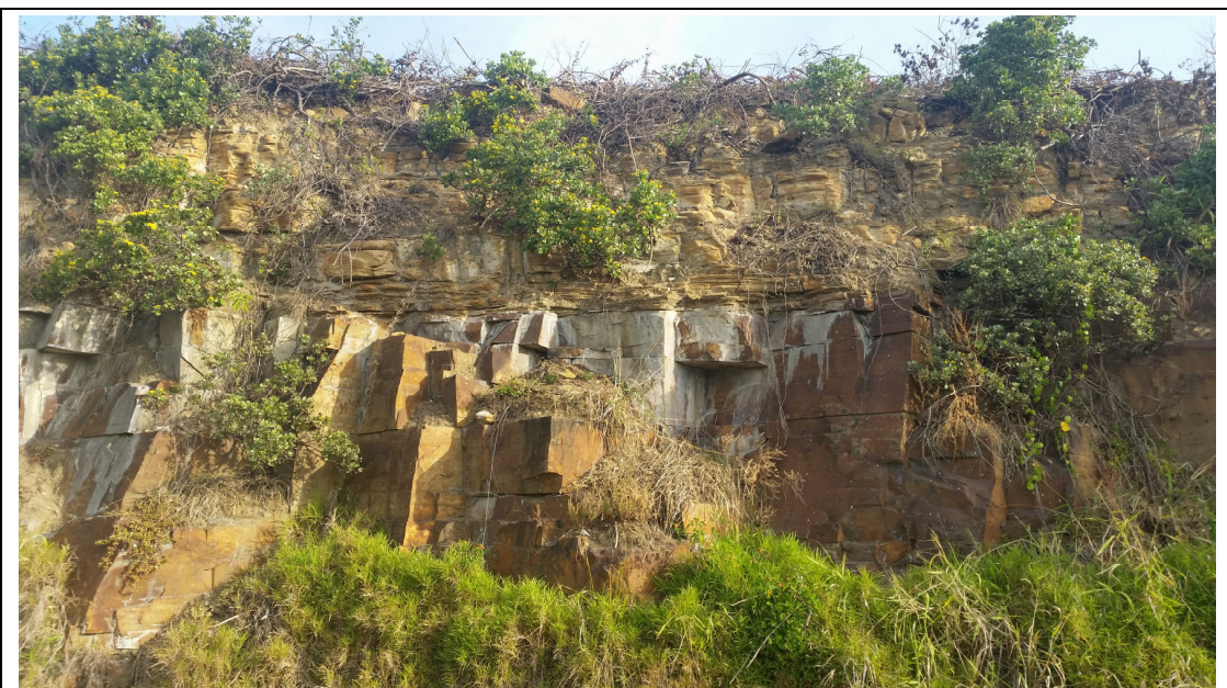
Photo 7: Visual indication of groundwater flow and seepage from horizontal bedding planes
