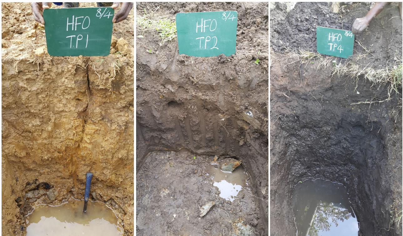
Photo 12: Groundwater seepage encountered in test pits
