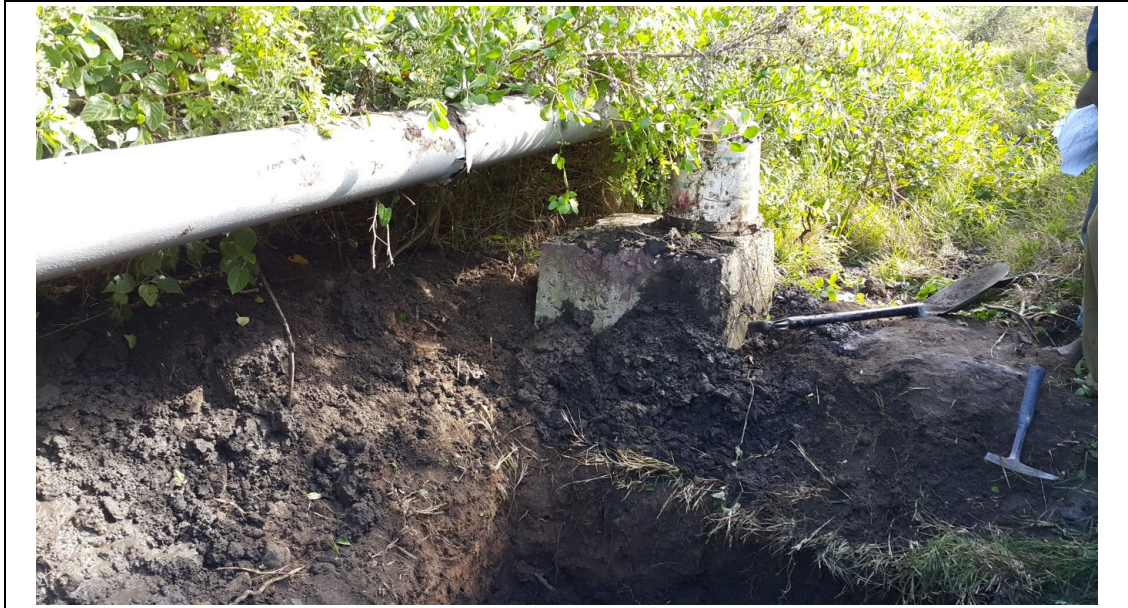
Photo 11: Position of test pit HFO – TP4
