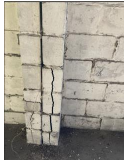
Figure 5: Structural Cracks
