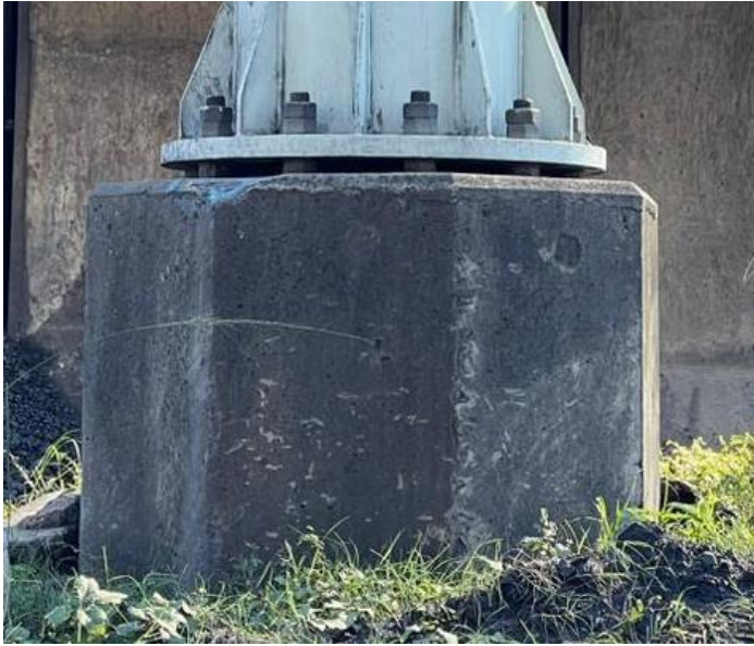
Figure 2: Spalling Concrete
