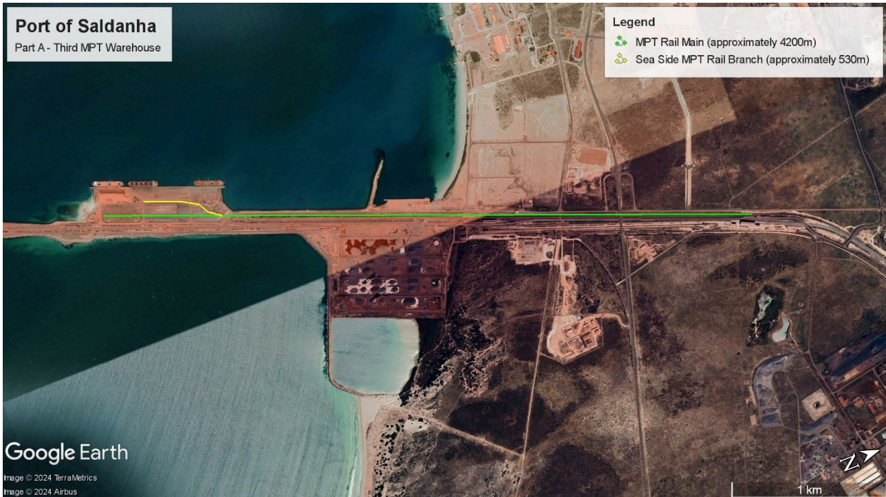
Figure 3: Upgrade of existing railway lines, approximately 6km extent, to 30 ton/axle load.
