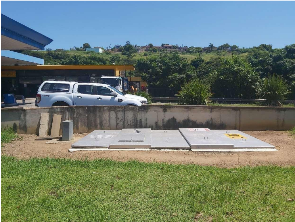
Figure 1: Sasol Filling Station, Demarcation Wall & TPL Block Valve Chamber
