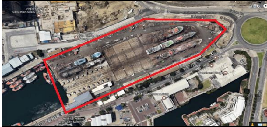
Figure 2. Overview of Syncrolift Dry Dock
