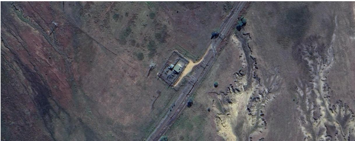
Pic 1. Distribution substation view and surrounding area where the substation is located
